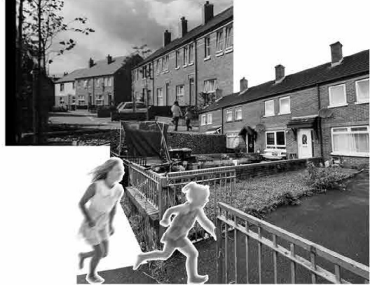
Character of the area remains. The shared service concept - there are no streets instead of pleasantly paved area is shared by the residents who houses are designed in a group or in a courtyard style.
