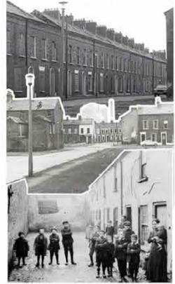
Donegall Pass was a district of well-paid artisans and small merchants by late-Victorian times. The housing no longer sufficient for the residents to have bathroom and a space for car.
