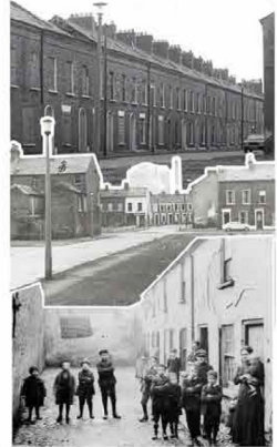
Donegall Pass was a district of well-paid artisans and small merchants by late-Victorian times. The housing no longer sufficient for the residents to have bathroom and a space for car.
